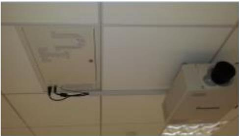
From the TEK 1201 in the podium to the receiver in the ceiling box only a single Cat 5e cable is required. This cable provides for both video and control of the system.
